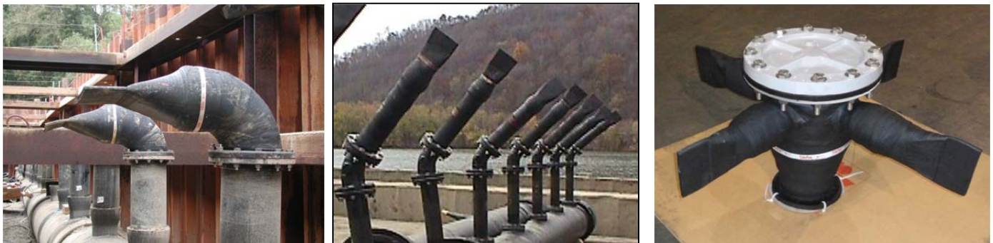
Figure 5 – Duckbill nozzles with integral wire-reinforced rubber elbows, risers, and 4-port rosette
