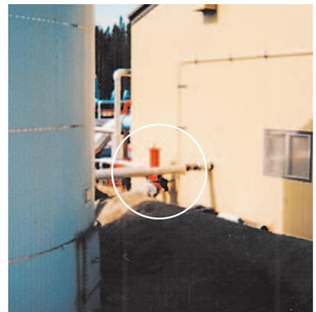
*Inlet separator tank to remove water and sand from field gas. Series 5200 maintains level control.*
