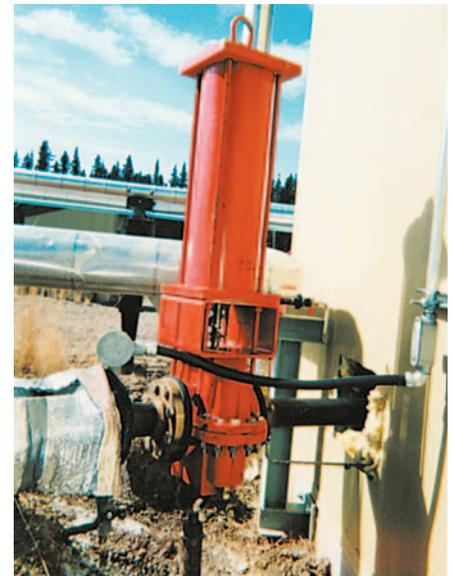
*Series 5200 fitted with spring-loaded, fail-closed actuator for tank level control.*
