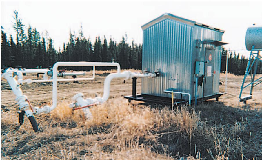
*Gas wells are controlled by a metering skid in remote areas of N.W. Canada.*
