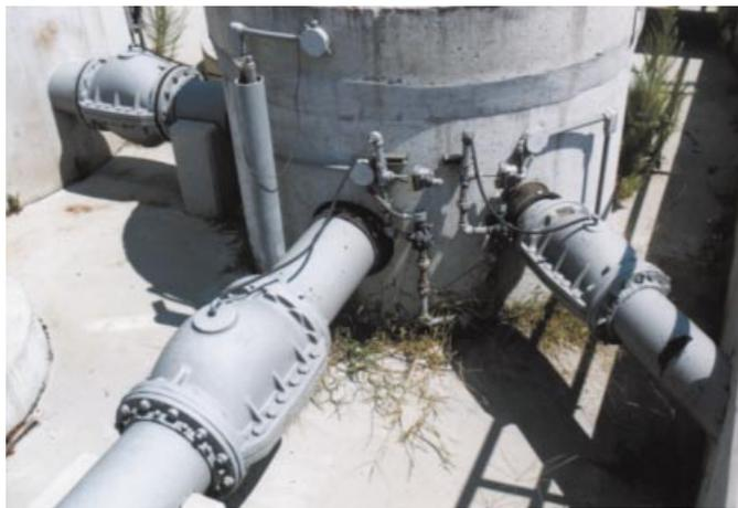
These Type A Pinch Valves are installed on a central column where influent is distributed to different settling and aeration tanks for treatment. The valves must contend with abrasive grit and raw sewage to provide accurate metering of the influent.
