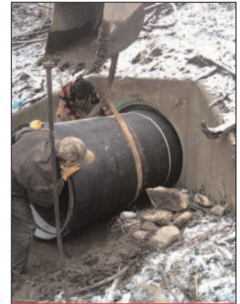
The CheckMate® Valve, being slid into the CSO pipe during installation.
