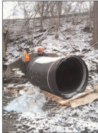
The 48" CheckMate® Inline Check Valve, prior to installation.
