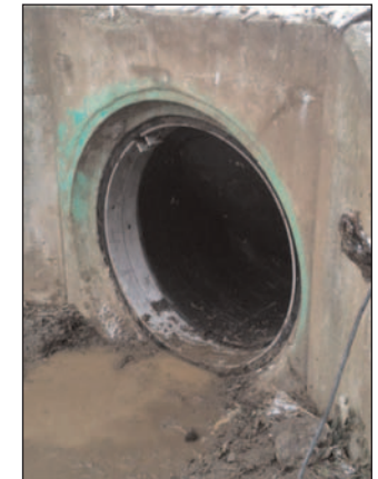
The CheckMate® Valve, after installation is completed.
