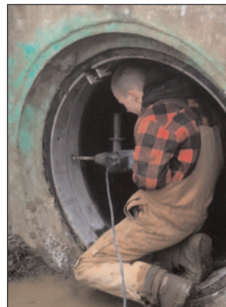
The 48" CheckMate® Valve, being clamped into place during installation.
