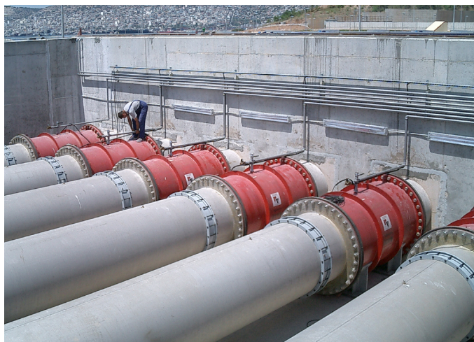
Eight 1200 mm Type A Megaflex pinch valves installed on the sludge distribution line at Psyttalia WWTP.
