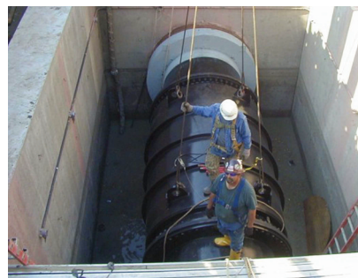
The 72" Type A Megaflex being installed in the interceptor vault.
