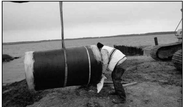
**STEP D:** Lubricate the valve and rubber adhesive strip surface. Slide valve into pipe. Ensure the area marked TOP is in the 12:00 position.
