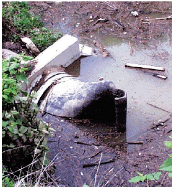
The curved bill of the TF-1 seals tightly around debris.
