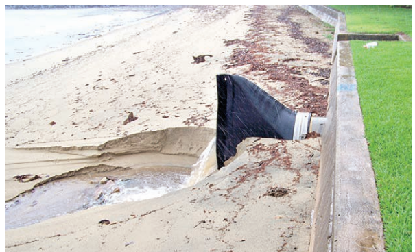
Views of Tideflex® TF-1 Check Valves installed along coastline. Note the curved bill design of the check valves does not hinder the valve's ability to open and flow in the sand.
