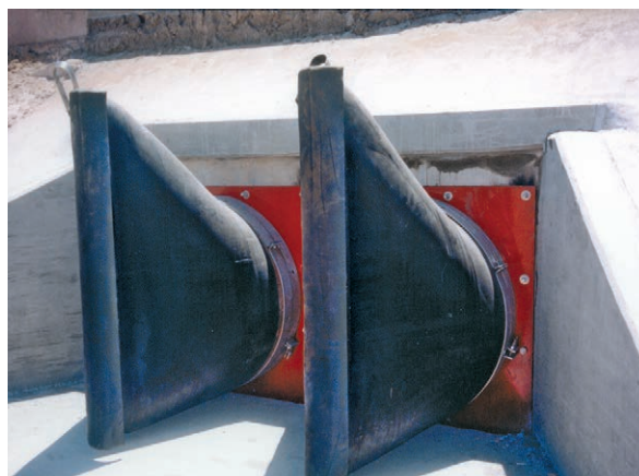
The TF-1 spine is at a greater angle than the TF-2, reducing the cantilever effects of water weight.
