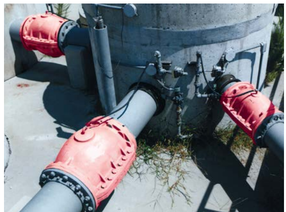
PAV Air-Actuated Pinch Valves (Type A) on a distribution column.
