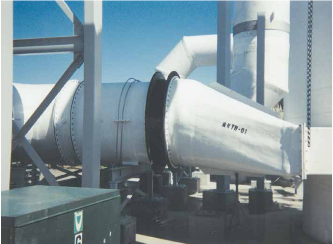
72" Redflex® Expansion Joint on air recovery system at a coal fired power plant.
