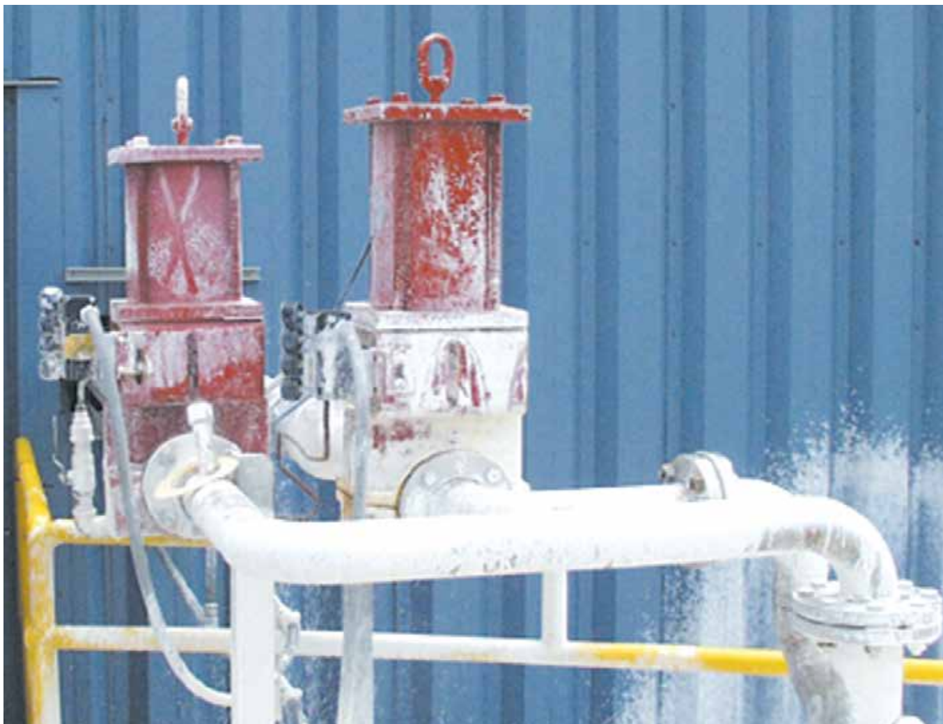
Series 5200 Control Valves with cone sleeves on lime slurry.
