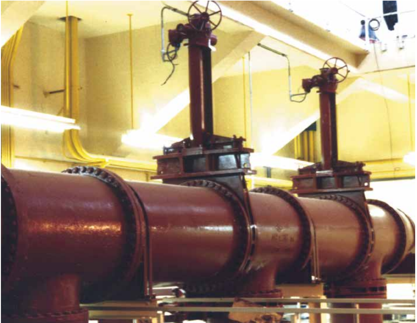
54" Knife Gate Valves on raw water intake system.
