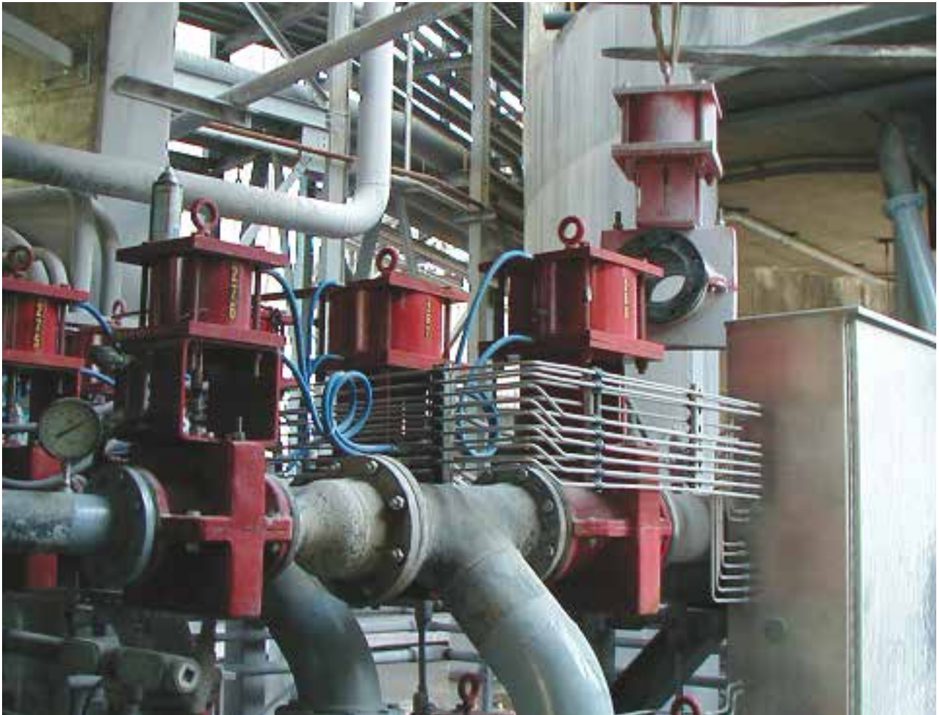
Series 5200 Control Valves being installed at a power plant.
