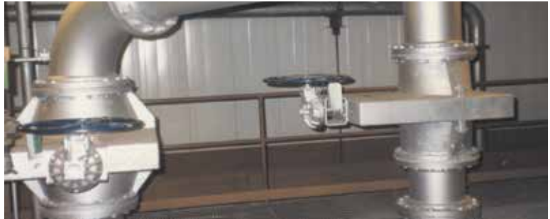
Series 75 Manual Pinch Valves on lime recirculation line.
