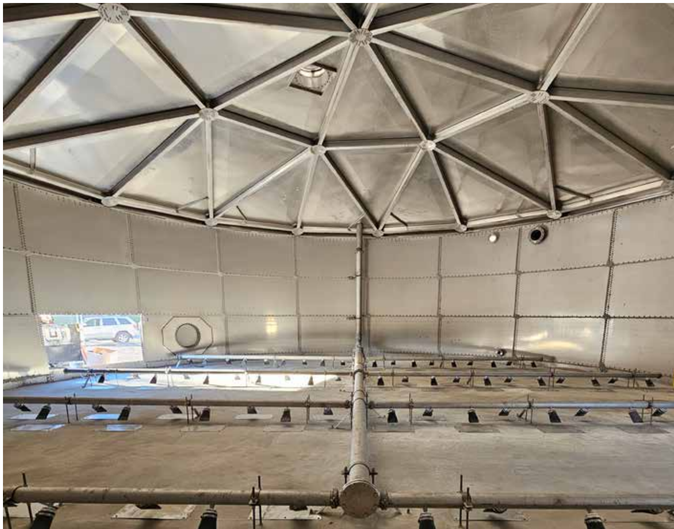
Tideflex® Aeration and Mixing System installed inside a tank.
