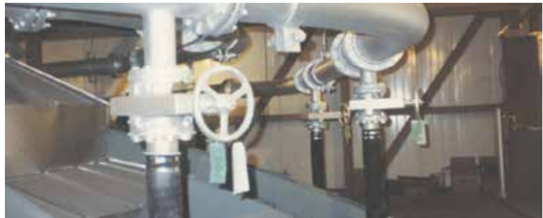
Series 75 Manual Pinch Valves on control spray nozzles.
