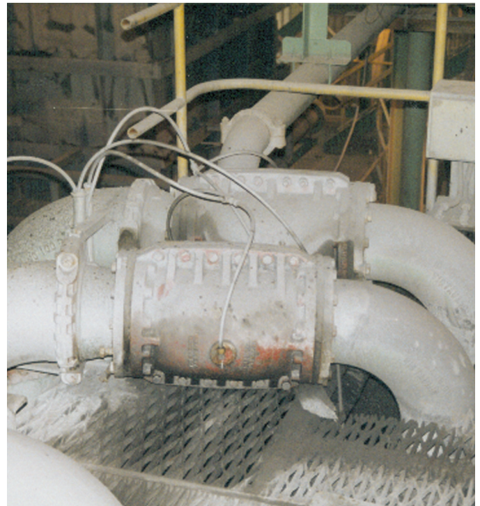
PVA - Type A Air-Actuated Pinch Valves being used on lime slurry control.
