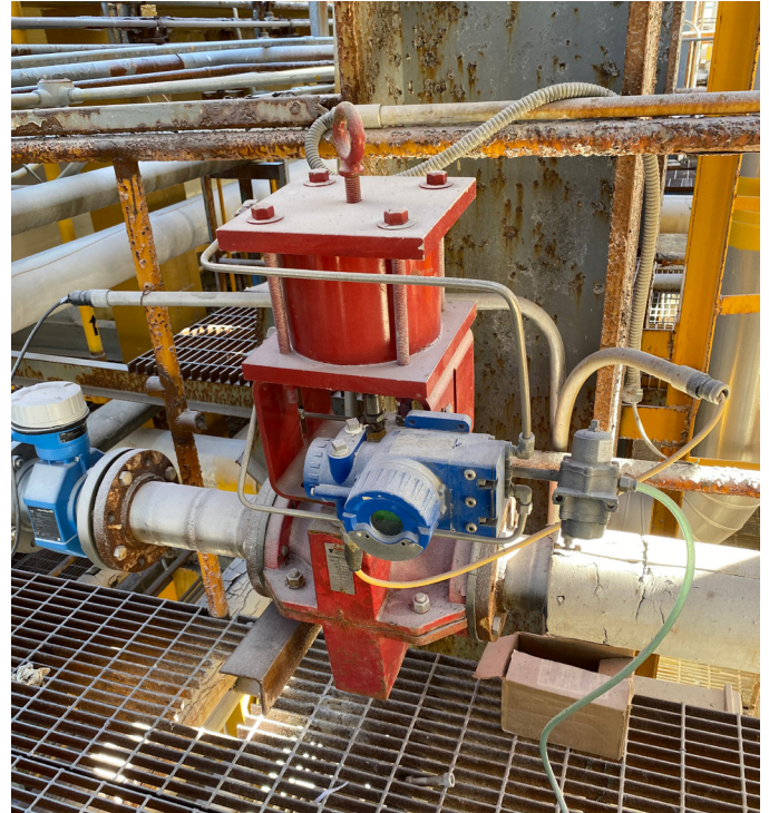
PCV - Series 5200 Control Pinch Valve used for level control in a drying process at a sodium sulfate mine.
