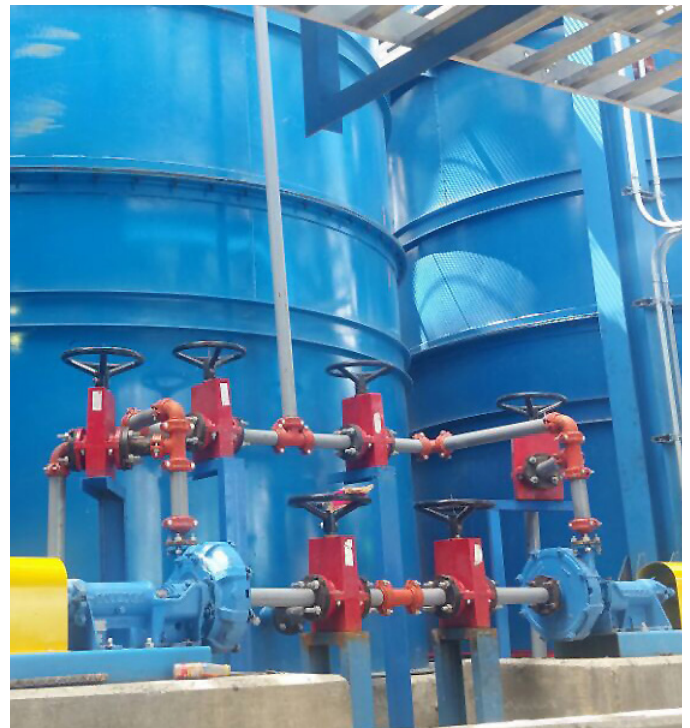
PVM - Series 75 Manual Pinch Valves on chemical reactor tanks at a copper mine.
