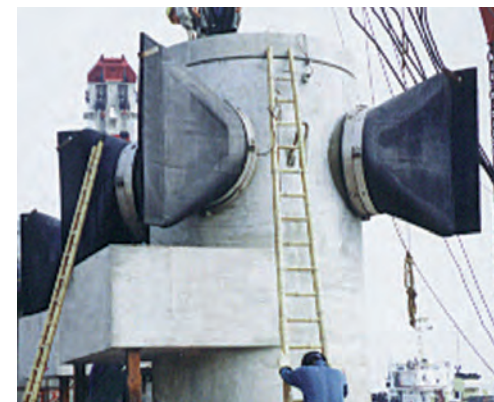
(12) 1,050mm Tideflex® Diffuser Valves installed on emergency outfall in Hong Kong.
