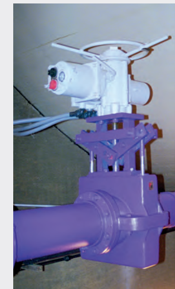
Electrically Actuated Series 5400E controls digester sludge accurately and requires no maintenance.
