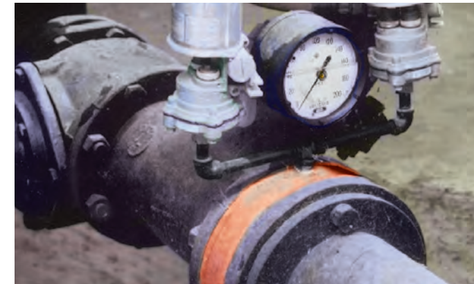
Red Valve Pressure Sensors are used with pressure gauges and transmitters, sending signals to protect pumps from running dry.
