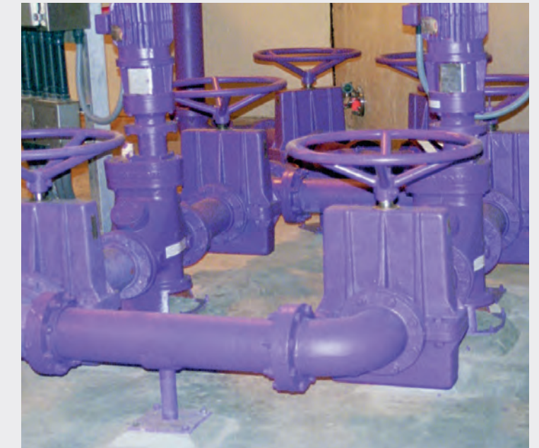
Manual Series 75 Pinch Valves on reactivated sludge provide years of maintenance-free operation.
