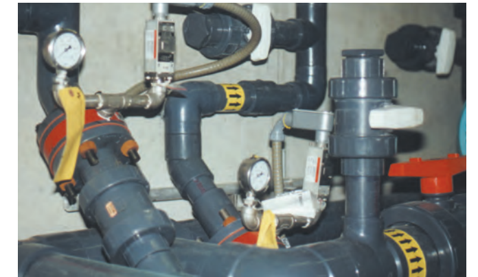
Red Valve Pressure Sensors used for accurate reading of polymer feed system.
