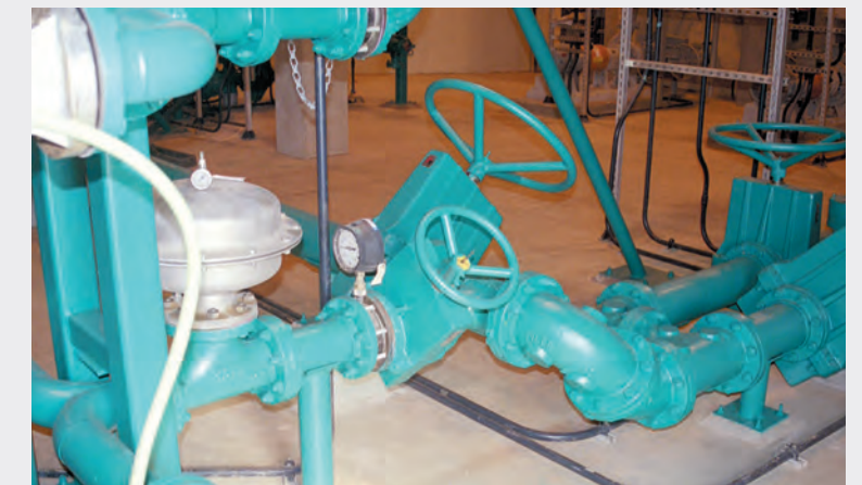
Series 75 and Pressure Sensors with Hypalon Sleeves are the ideal choice for sodium hypochloride and other corrosive chemical additives. The sleeve is the only wetted part, providing a long-term, corrosion-resistant service life.
