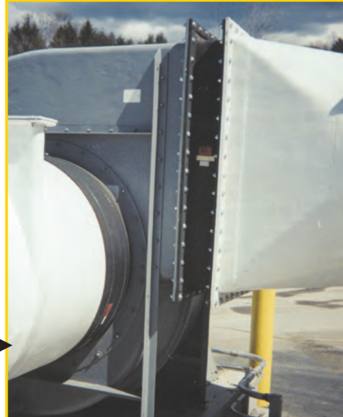
Circular 72-inch ducting joints on an air-recovery system at a coal-fired power plant
