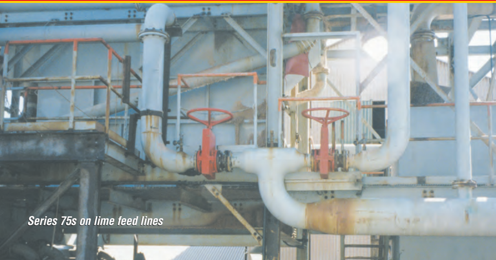
Fail-closed control valves on ash
