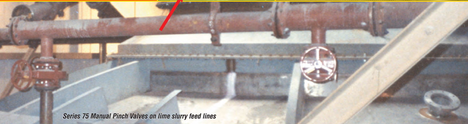
Large-diameter Series 75 Manual Pinch Valves on a lime-recirculation line
