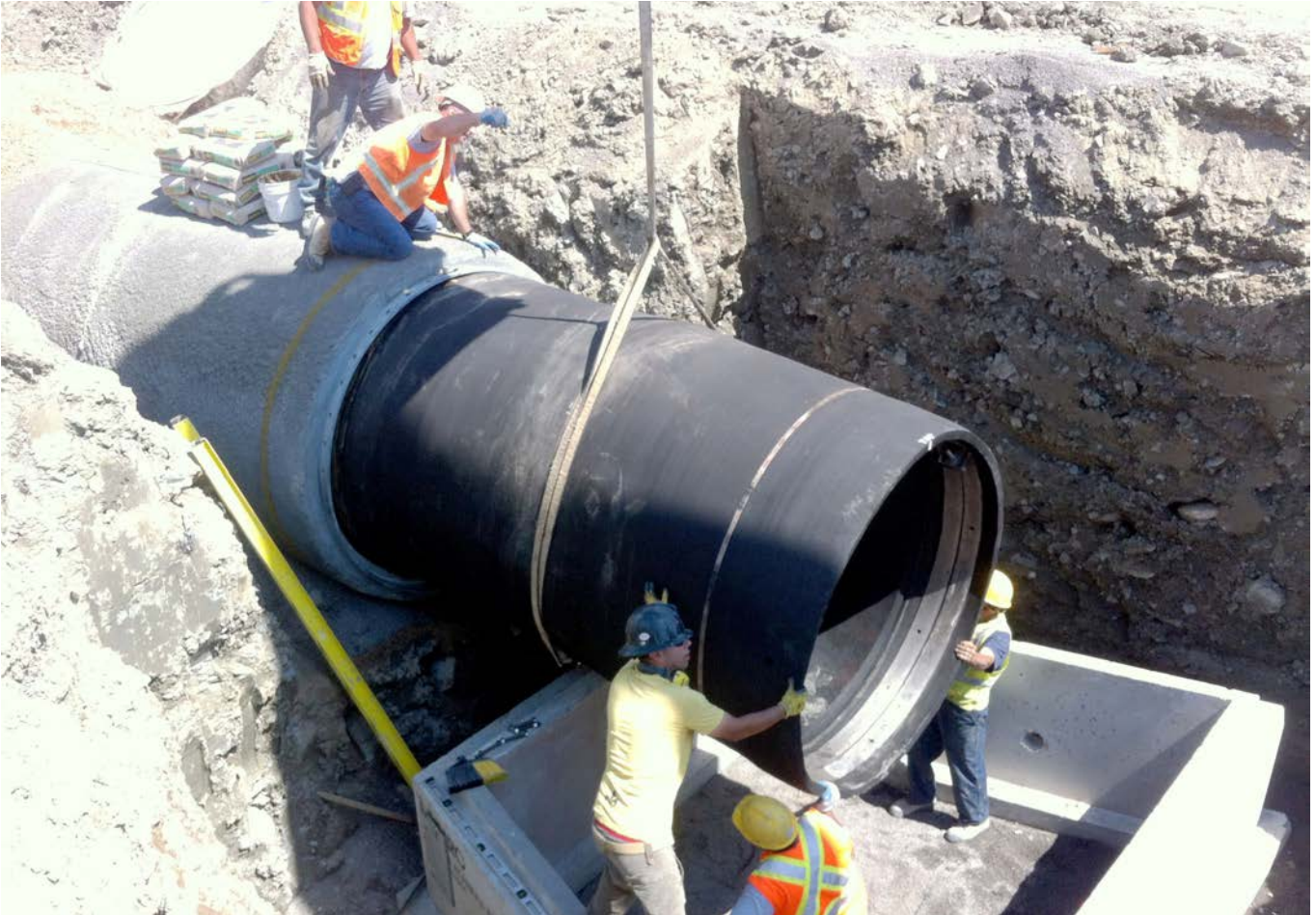
CMU CheckMate UltraFlex® In-Line Check Valves provide backflow prevention and odor control.
