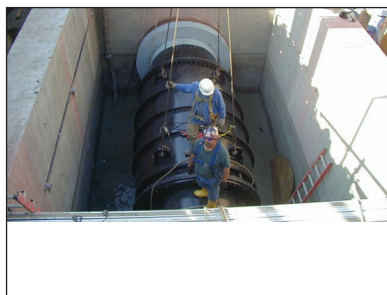
72" Type A Megaflex Valve being installed in an interceptor vault to control waste water flow for the city of Indianapolis.
