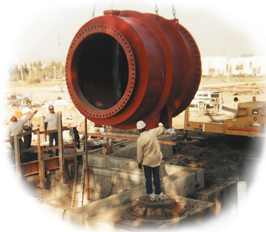
This 30" Series 5200E Electric Actuated Control Pinch Valve is installed in a waste water treatment plant in Georgia. The flexible elastomer sleeve can seal on solids, such as branches, bottles, and other storm-water debris, with-out damaging the valve. The Series 5200E is ideal for on/off control in this service.
