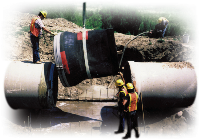
This 54" Series 37 Inline Check Valve is being installed in a concrete pipeline. The Series 37 is designed to fit within the pipe I.D., eliminating the need for valve bodies and simplifying installation.
