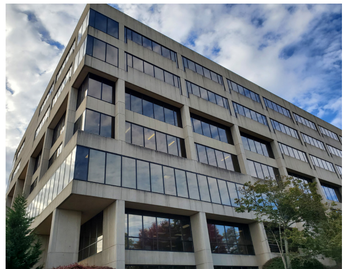
Red Valve's headquarters in Pennsylvania.
