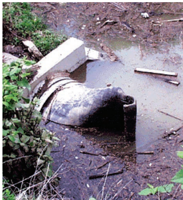
The curved bill of the TF-1 seals tightly around debris.
