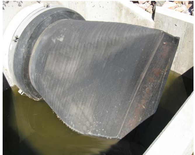
A 20" check valve with a 30" cuff, built by another check valve manufacturer. This was passed off as a 30" check valve.
