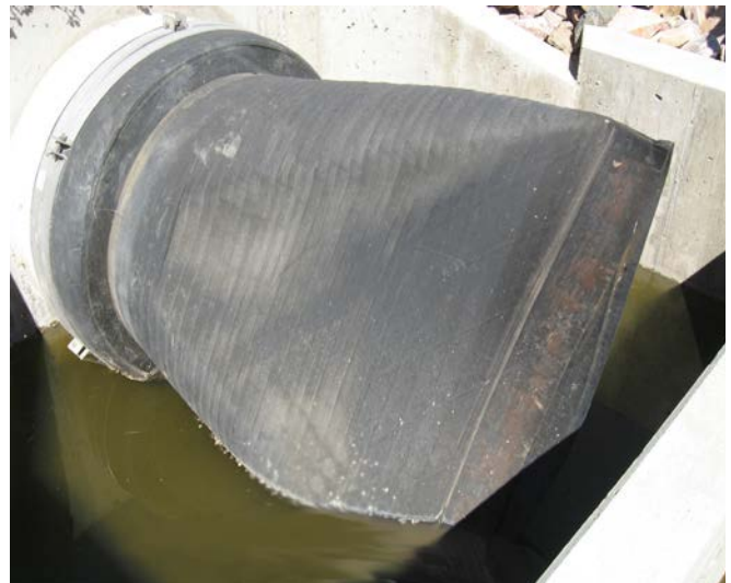
A 20" check valve with a 30" cuff, built by another check valve manufacturer. This was passed off as a 30" check valve.
