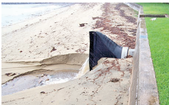
Views of Tideflex® TF-1 Check Valves installed along coastline. Note the curved bill design of the check valves does not hinder the valve's ability to open and flow in the sand.
