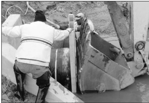
Pallet Push method for installing CheckMate® Valve
