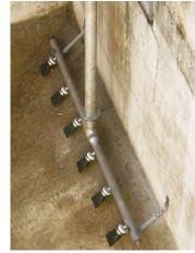
Holding raw wastewater in a quiescent chamber will also result in stratification and separation of floatable solids (fats, oils & grease - FOG). These materials will remain floating on the surface because most pumping systems have a low level shut-off point and cannot remove the entire contents of the storage wetwell. This can result in a requirement for installing mechanical removal equipment or implementing manual removal practices.
