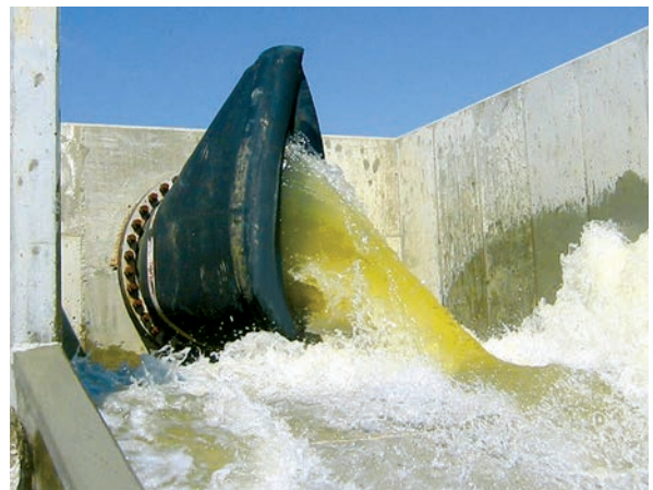
The increased driving head of a TF-1 Check Valve improves flow capacity.
