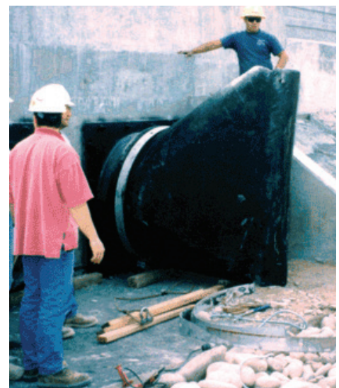
The eccentric TF-1 Check Valve is designed to accommodate installations with little ground clearance.
