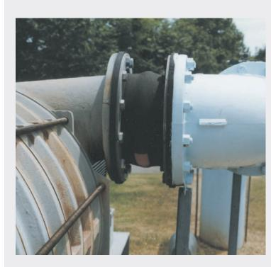
**Redflex® Expansion Joints** absorb vibration and compensate for pipe misalignment and movement. They help alleviate piping stress and reduce noise. Red Valve offers flanged and slip-on connections, single or multiple arches and a range of elastomers to meet process conditions, including Teflon®-lined joints for severely corrosive applications.
