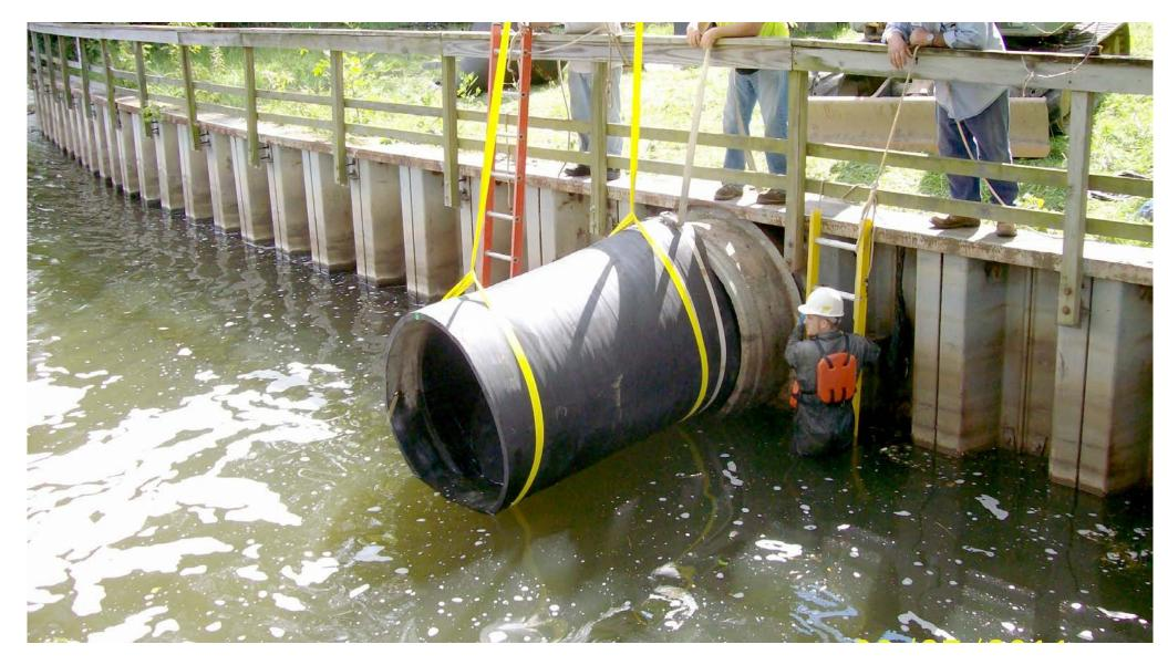
Tideflex® Check Valves and CheckMate® In-Line Check Valves are proven, reliable components in Effluent Diffuser Systems designed to increase dispersion and eliminate backflow. During an overflow event, or final discharge, flow passes freely across the valve, with the benefit of preventing unwanted river, bay or ocean water from entering the collection system.
