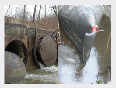
**Problem:** Traditional flap gate valves get stuck open, allowing millions of gallons of water to go back into systems or treatment plants for re-treating.
