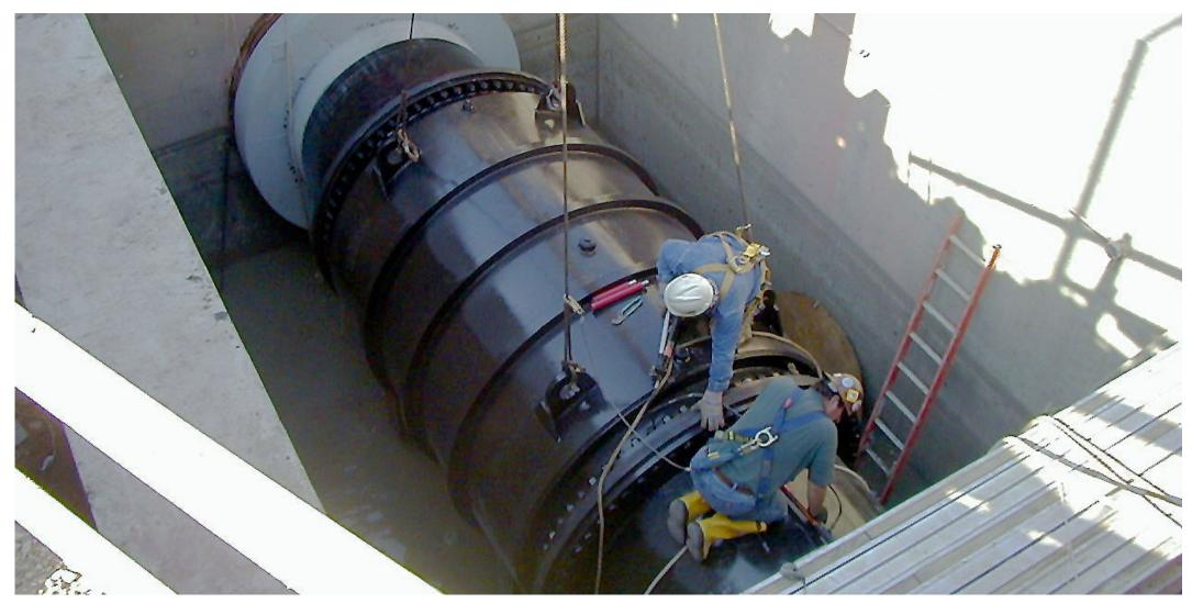
One of the most challenging applications for any municipality is influent flow control. Red Valve's unique products such as the Type A Megaflex Valve are specifically designed to store, control and isolate stormwater flows within collection system piping. This control strategy minimizes combined sewer overflow volume and frequency.
