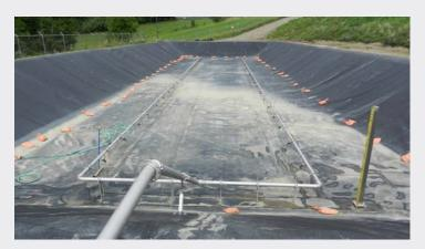
Simple and efficient Tideflex<sup>®</sup> Check Valves, used as mixing and aeration nozzles, are the perfect solution for preventing stagnation in stormwater storage and detention basins.
