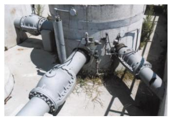
These Type A Pinch Valves are installed on a central column where influent is distributed to different settling and æration tarks for treatment. The valves must contend with abrasive grit and raw sewage to provide accurate metering of the influent.
