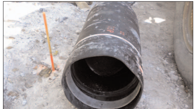
The CheckMate® Inline Check Valve, prior to installation.
