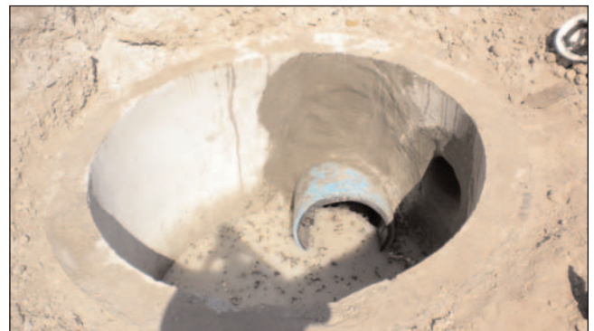
The installed CheckMate® Valve, holding back water.
