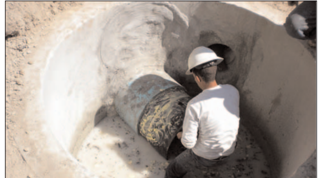
The CheckMate® Valve being installed into the box culvert.
