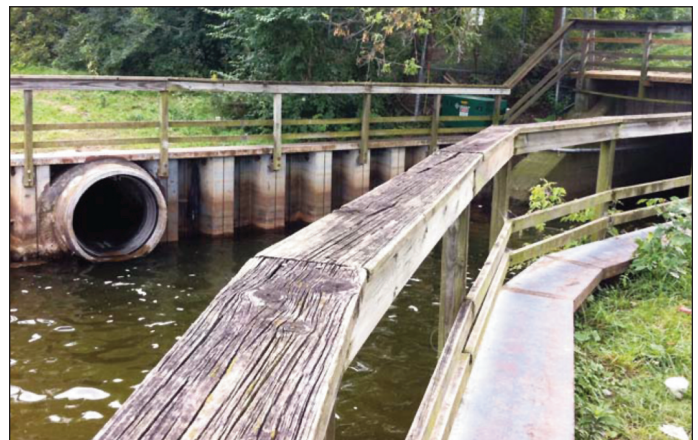
48" Tideflex CheckMate® Installed on Storm Sewer at Allen Creek Drain
