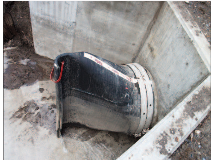
A Tideflex® TF-1 Check Valve installed on the River Barrow to protect Carlow from flooding.
